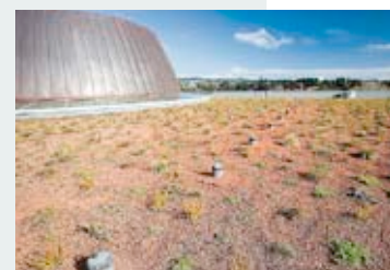
After installation: The native plants are designed to be low and slow-growing
