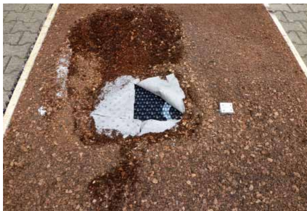
No effects of the fire were observed on the filter sheet or the drainage element.
