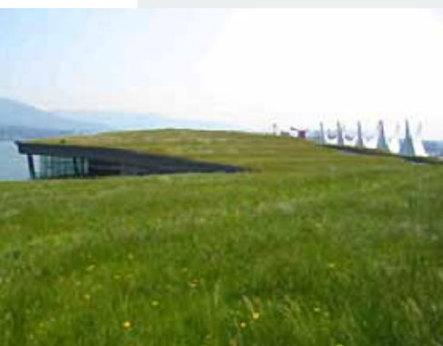
The Vancouver Convention Centre Roof Looking North and East
