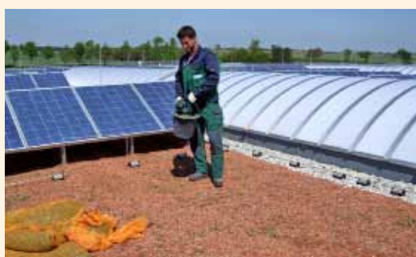
Sedum cuttings are used for the plantings
