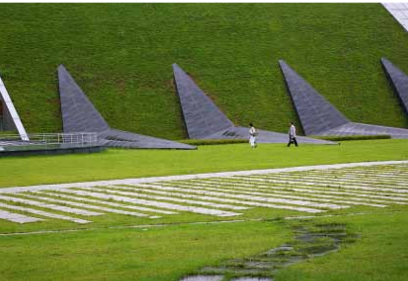
2nd place award winning project of the 2nd Korea Green Roof Award in 2010. The whole green area shown in the photo covers library buildings and digital library below.
