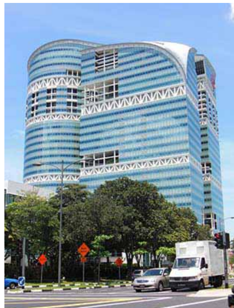
Photo shows the 3 towers of Fusionopolis
