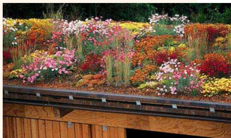
Summer look of the biodiverse roof in Schopfloch
