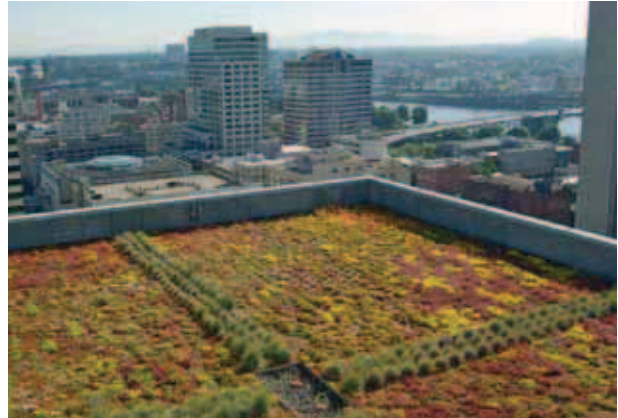
A City of Portland building with an ecoroof
