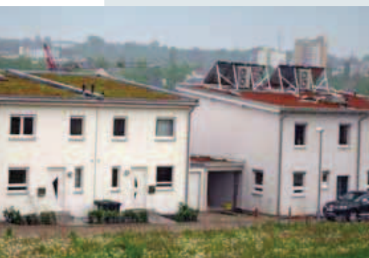
Green roofs and renewable energies are mandatory at the building site Hohlgrabenacker.
