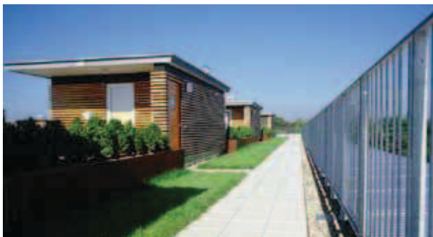
Easy access to the garden via the rooftop studio
