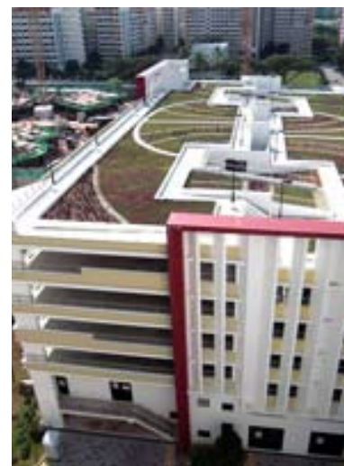
Singapore's first, large scale, extensive-type green roof on top of the MSCP's at Sengkang East Avenue (left, middle) and at Tah Ching Road (right).
