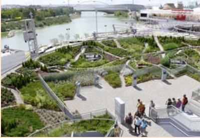
The lush vegetation, intersected by narrow strips of gravel, highlights the image of the rooftop garden
