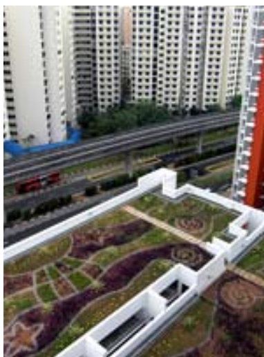
Singapore's first, large scale, extensive-type green roof on top of the MSCP's at Sengkang East Avenue (left, middle) and at Tah Ching Road (right).
