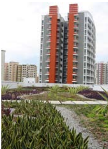
Singapore's first, large scale, extensive-type green roof on top of the MSCP's at Sengkang East Avenue (left, middle) and at Tah Ching Road (right).
